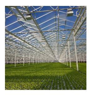
destined for a huge 20,000 m² greenhouse installation as part of a greenhouse extension project that will boost the total cultivation area to 49,000 m² at the site of a major Belgian lettuce grower using a unique experimental process, whereby the plants move slowly through the greenhouse on a conveyor beneath the LED lights. Taking 5-6 weeks to complete the journey, the lettuces are harvested at the end when fully grown.
